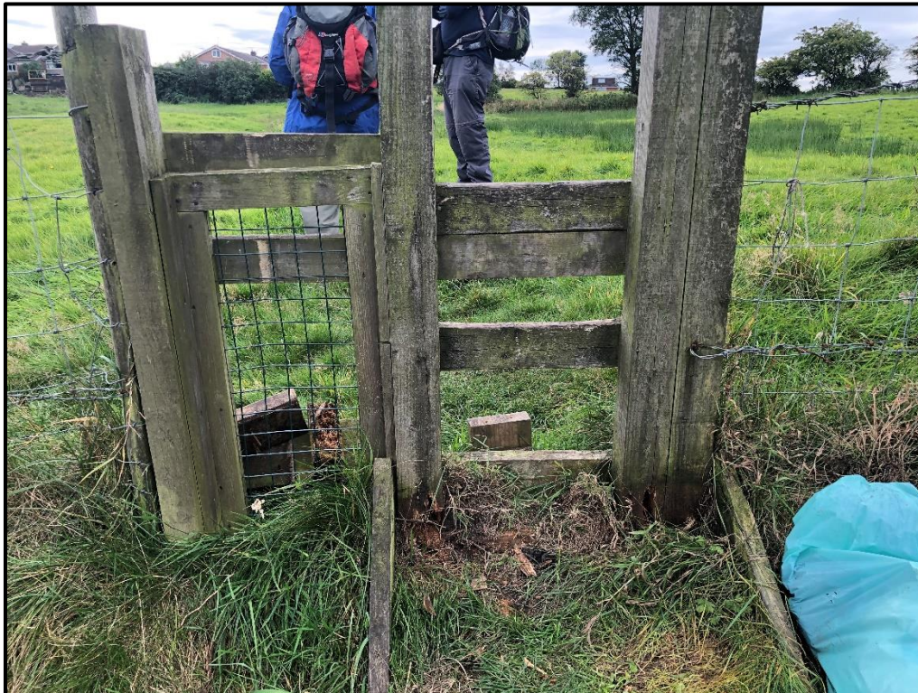
Footpath 79 [Crompton Circuit] on Samuel Lane, High Crompton. Step stile broken & top step riser rotted away.
